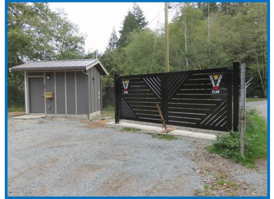
New Electronic Gate (not activated yet)
